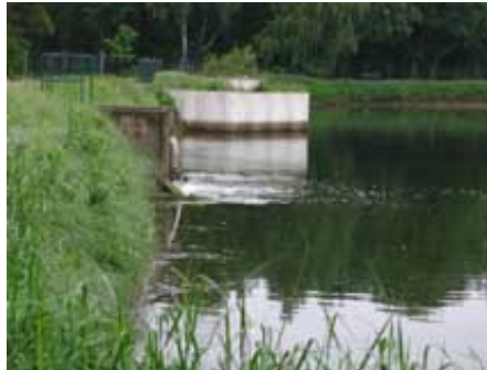
Artificial recharge pond in Tegel
