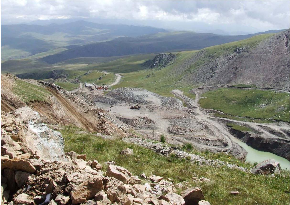
Partial view of the Solton Sary Gold-mine. Photography: Dörre, 2016
