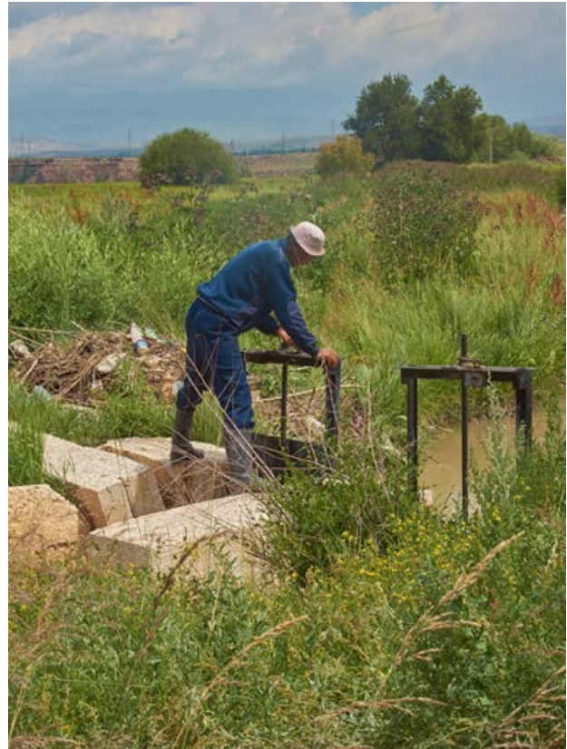
Fig. 3: Flow rate regulation at the gate of the Big Naryn Canal. Photography: Marx, 2016
