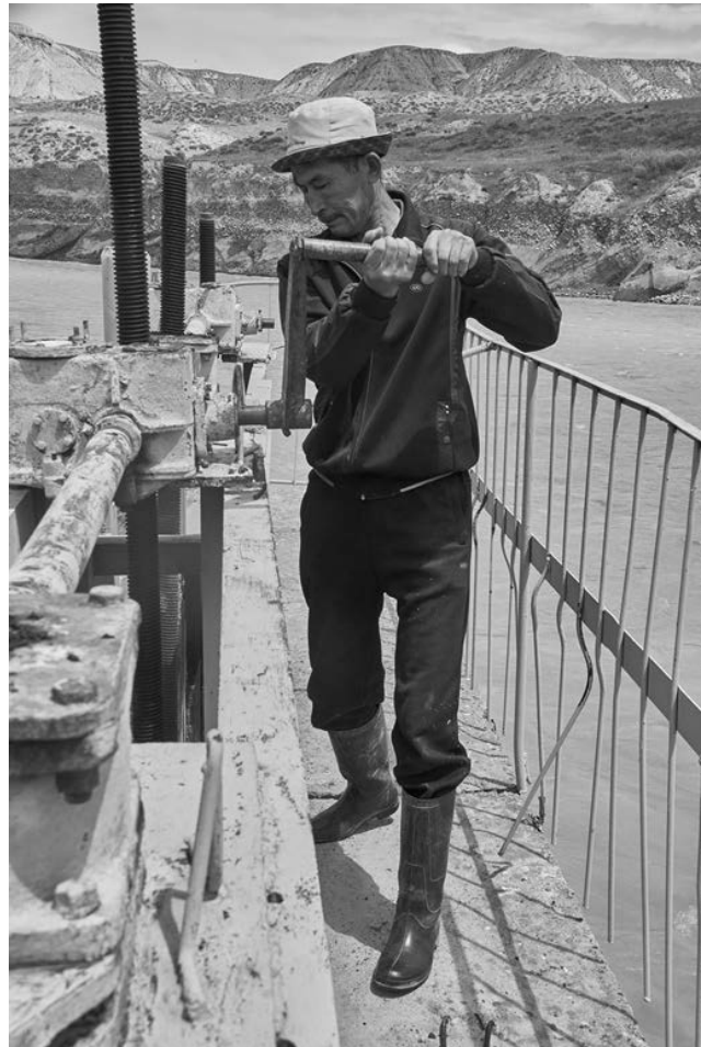
Fig. 6: Murab, opening the main gate at the Naryn River. Photography: Marx, 2016
